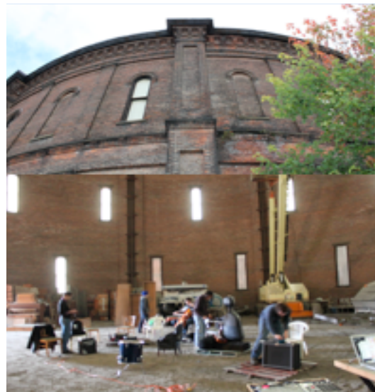
Figure 14 - Interior and Exterior of the Troy Gasholder House
